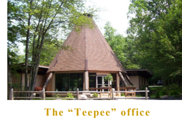
The "Teepee" office
