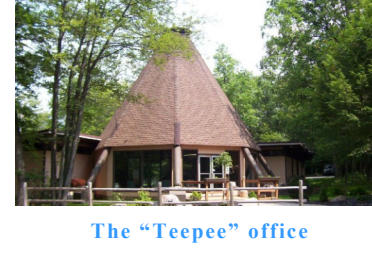
The "Teepee" office
