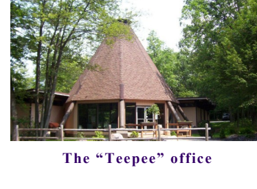
The "Teepee" office
