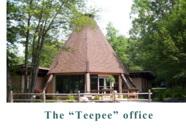
The "Teepee" office
