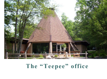
The "Teepee" office
